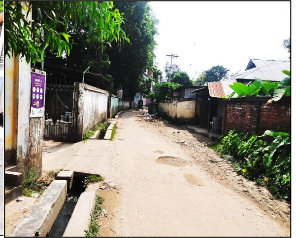
Drain-01, Madhupur Paurashava
