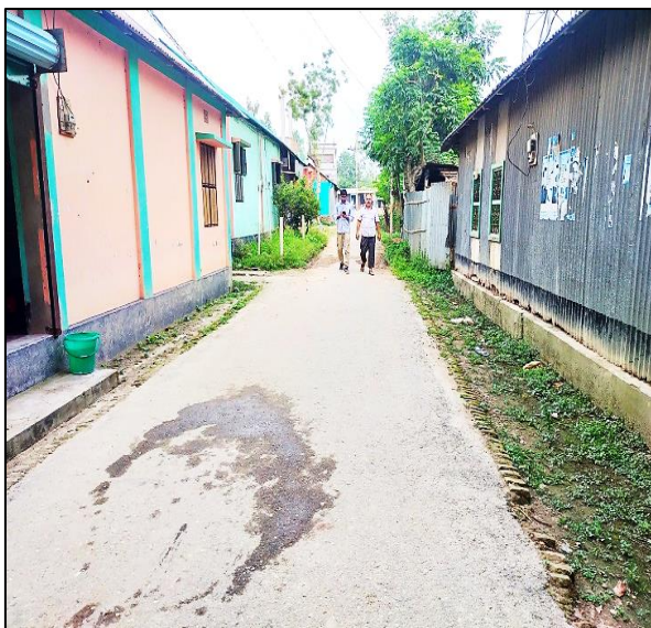
Drain-04, Madhupur Paurashava
