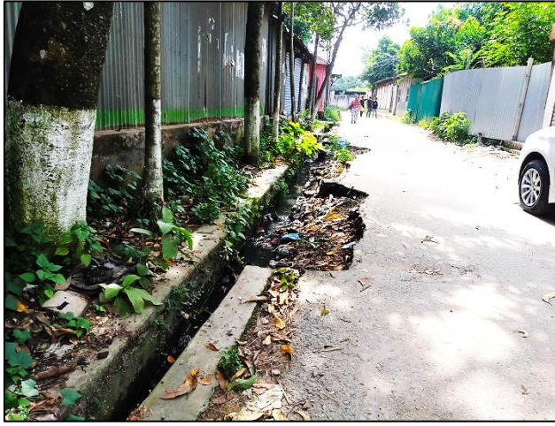
Drain-01, Madhupur Paurashava
