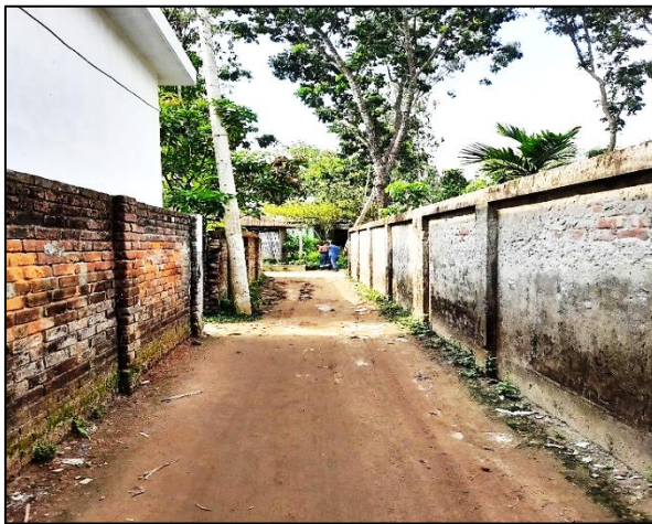
Drain-02, Madhupur Paurashava
