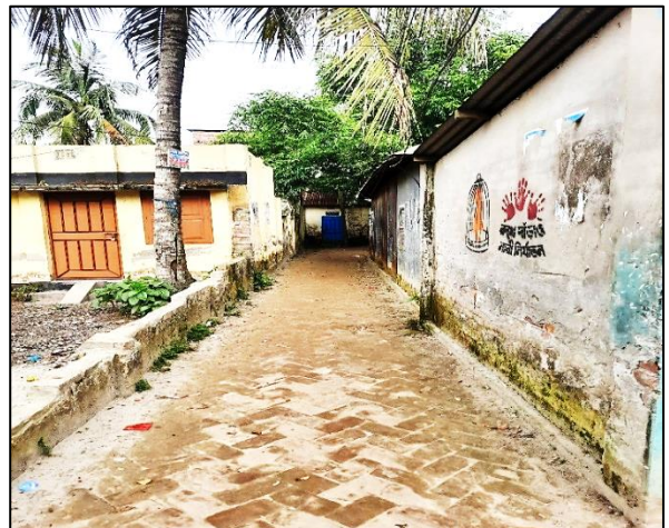
Drain-02, Madhupur Paurashava
